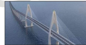
● Brunei cross-sea bridge project
