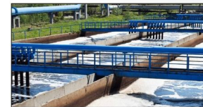
● Kuwait sewage treatment project
